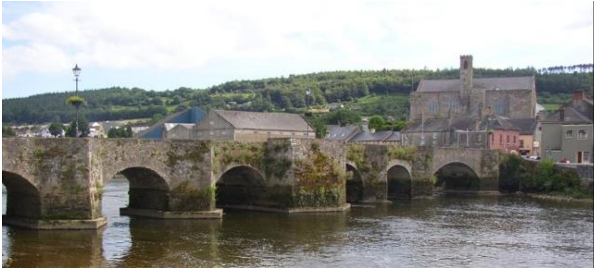
Figure 48 The Old Bridge across the Suir in Carrick on Suir, looking south towards CarrickBeg.
